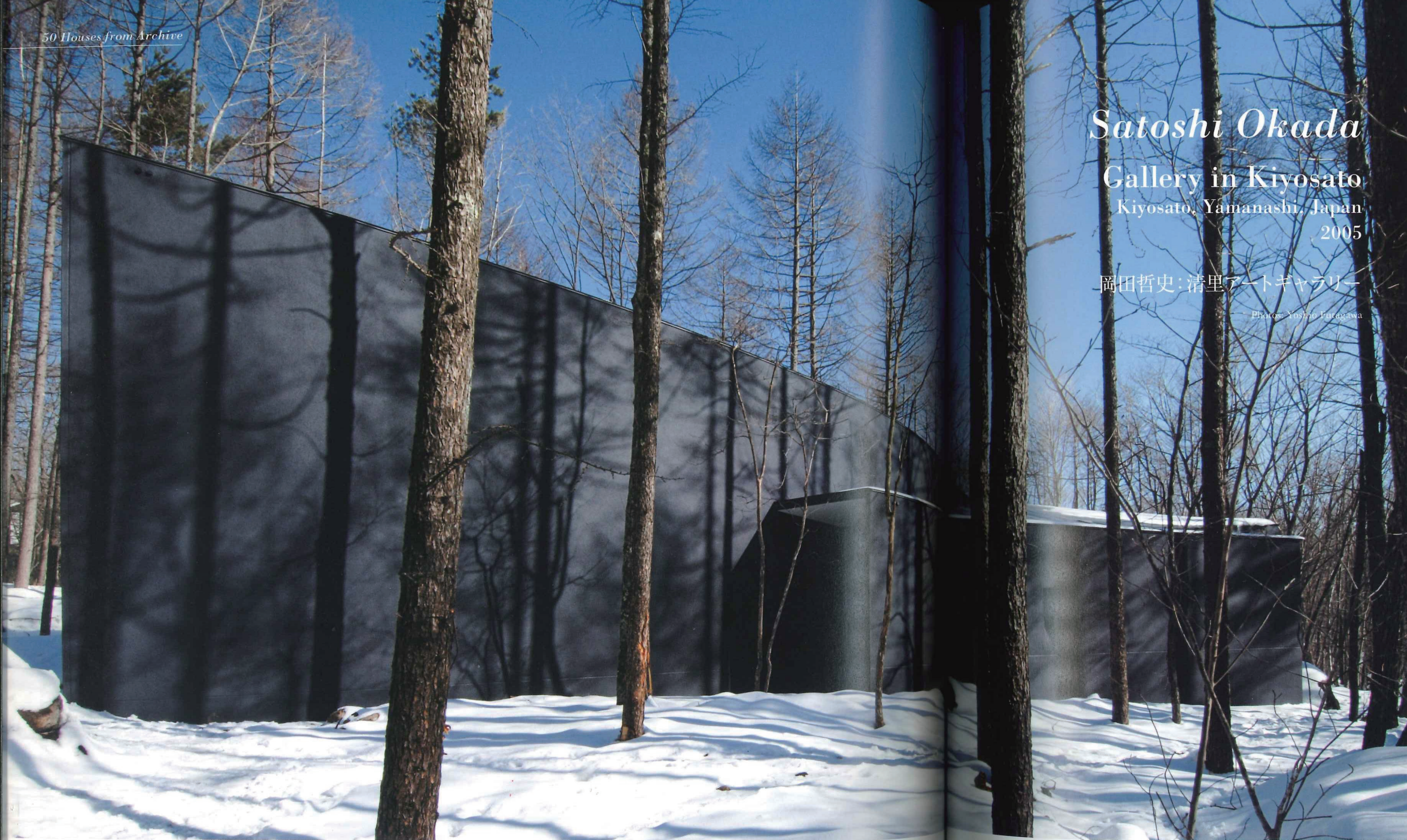
Overall view from south 南側全景
