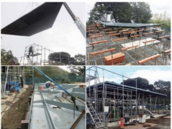
建築結構建造過程 THE PROCESS OF BUILDING CONSTRUCTION
